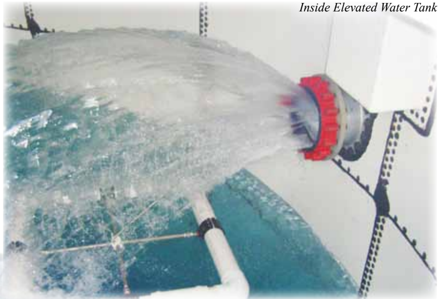
Inside Elevated Water Tank
